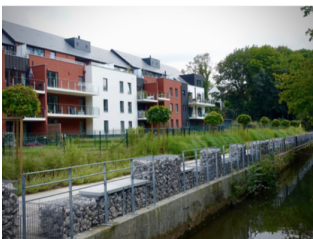
Ginkgo I Mont Saint Guibert, Belgium Former paper mill
